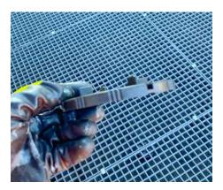
'MacroMesh' FRP grating installation using C-Clips and rubber spacer pads
